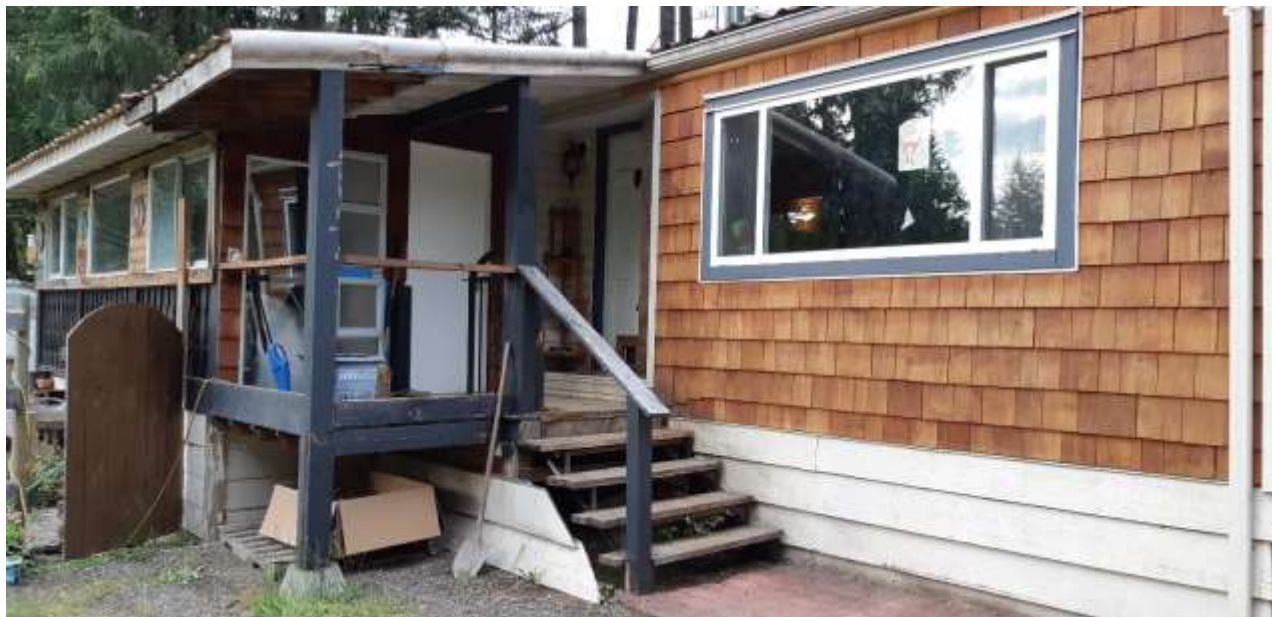
Figure 5: Subject Mobile Home with Front Porch (Front Porch will be Moved along with the Mobile Home Back Deck and Solarium will be Removed)
